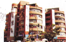
SHRI RAM TOWER
